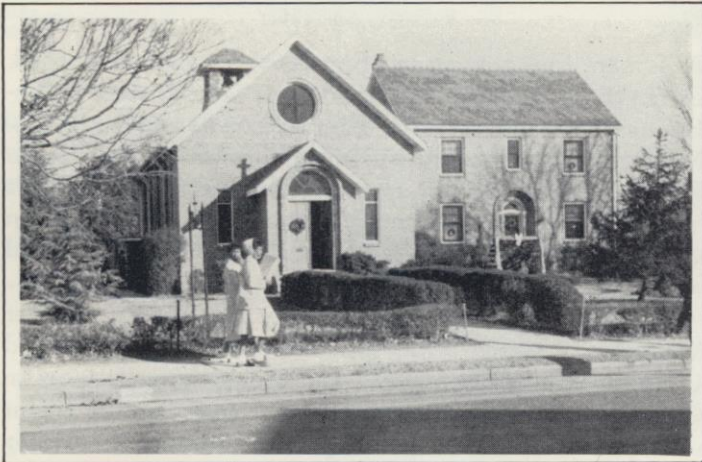
Church and rectory stand side by side on what was once a weed-covered field in North Carolina.
